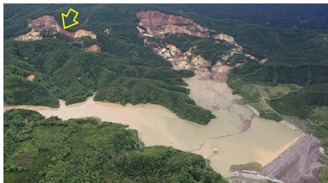
Photograph 2 Typical landslide in a reservoir rim
